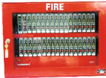
Conventional Fire Alarm Panel
